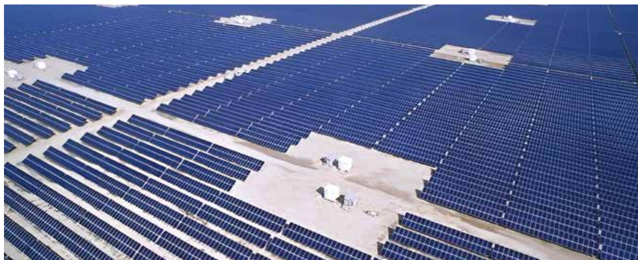
04 Utility Project in Pakistan 900MW PV Plant
