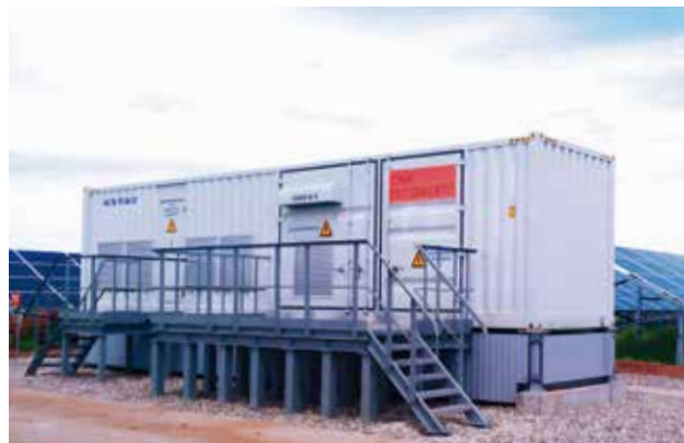
02 Utility Project in Russian 300MW PV Plant
