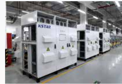
PV Assembly Workshop
